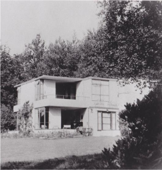
Sun House was altered substantially in the 1970's by Kathy and Gerry Green - the balconies were filled in and the concrete flat roof lies beneath a new tiled roof. It was completely changed
