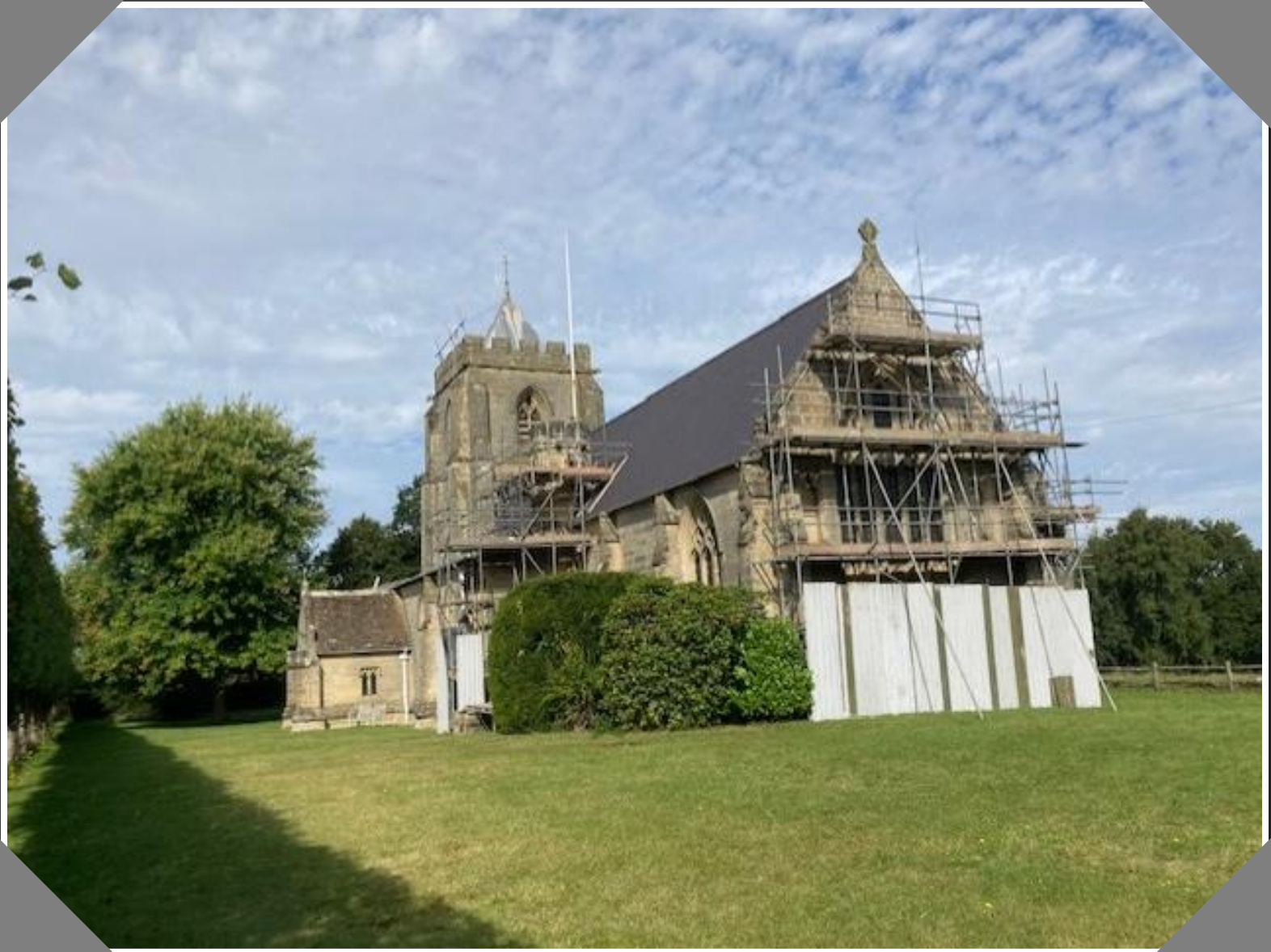
All Saints church's stained-glass windows being restored
