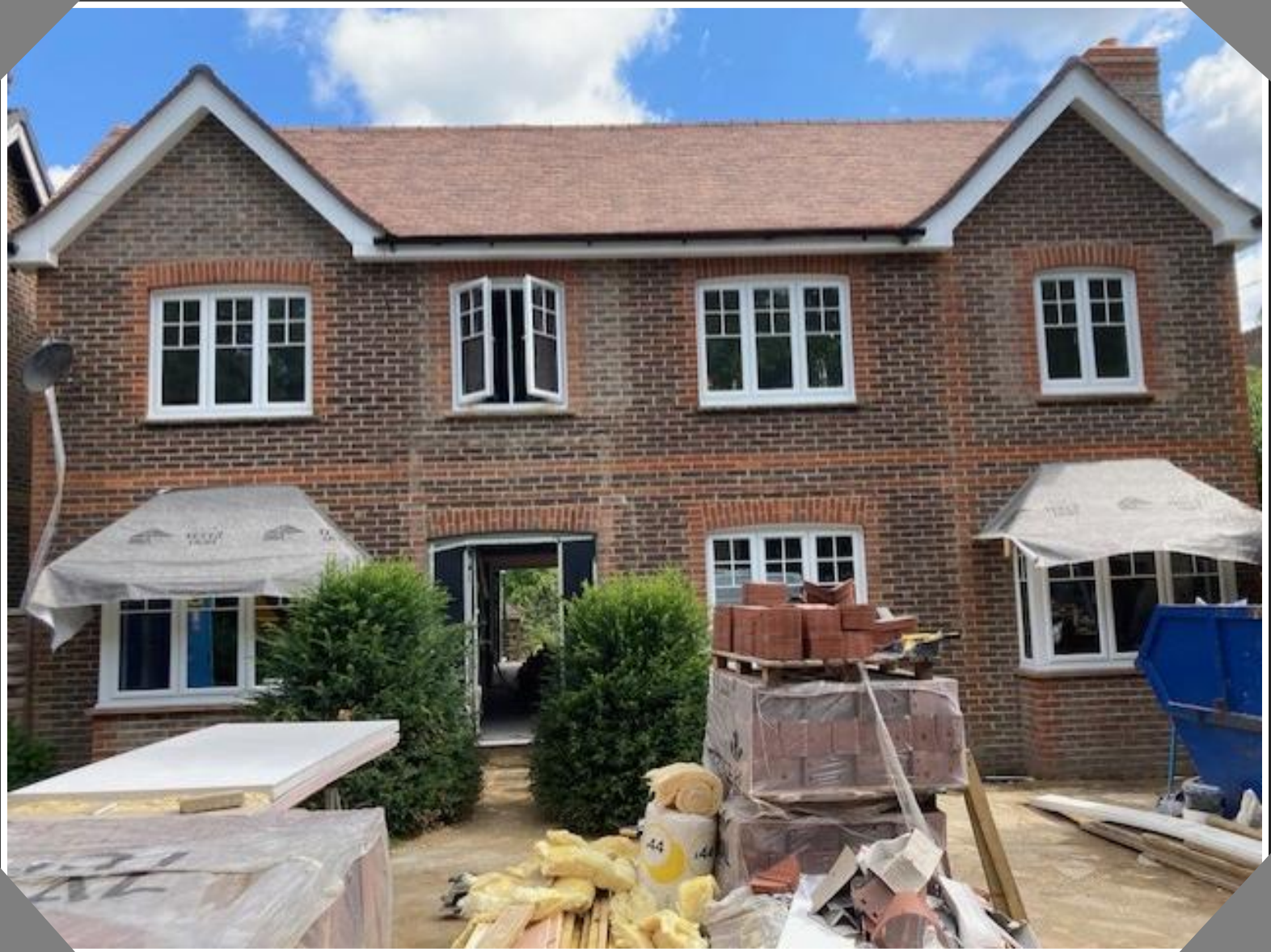
North View, Beaconsfield, Road, Chelwood Gate
